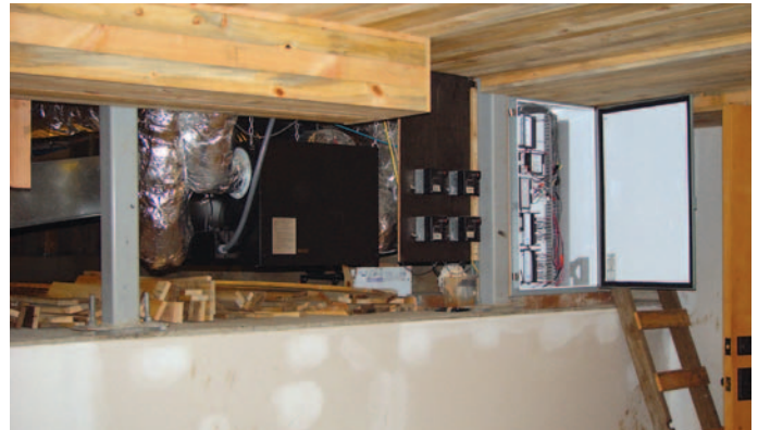
Ventilation and heating are delivered by a hydronic loop and pump; three energy recovery ventilators, or ERVs (left); and a direct digital control system. Right photo, the open controls cabinet with the Zone 1 ERV to the left. In between them are four relays used to operate three of the pumps and the heat pump.
