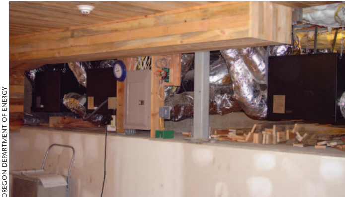
Ventilation and heating are delivered by a hydronic loop and pump; three energy recovery ventilators, or ERVs (left); and a direct digital control system. Right photo, the open controls cabinet with the Zone 1 ERV to the left. In between them are four relays used to operate three of the pumps and the heat pump.
